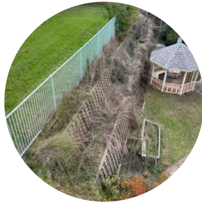
Existing cut on site including ~3.0m retaining wall
